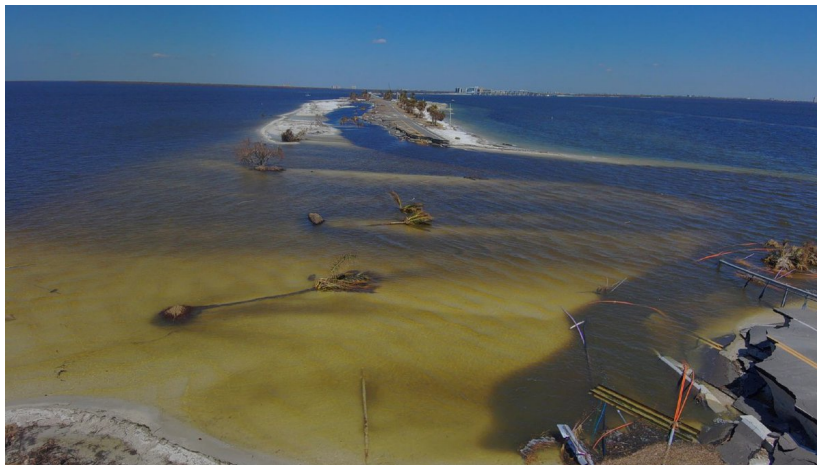
Figure 7. Hurricane Ian Damage to Sanibel Causeway (FDOT, 2022)
