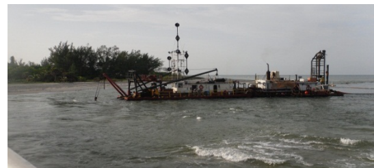
Dredge working a few yards off Blind Pass Bridge on Aug. 7
