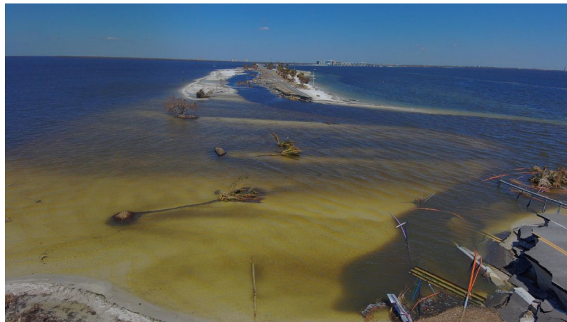
Figure 7. Hurricane Ian Damage to Sanibel Causeway (FDOT, 2022)
