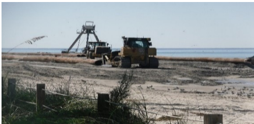
Nourishment construction during 2013-project
