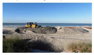
A bulldozer spreads the sand just pumped in from over 2 miles offshore
