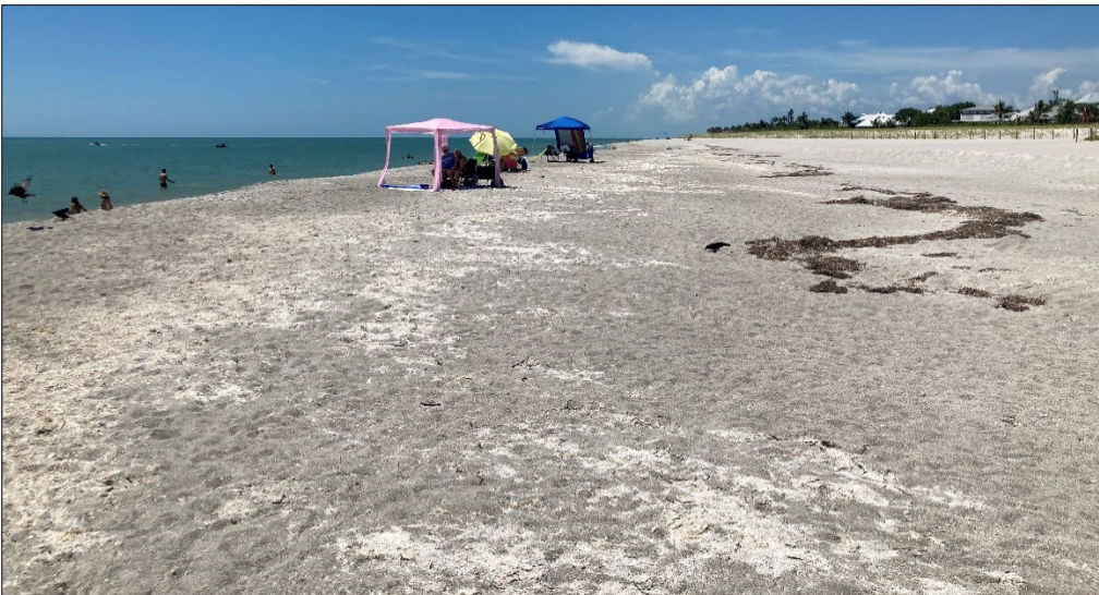
Figure 9. Northwest view of the wide sand beach and dune immediately north of the Blind Pass terminal groin.
