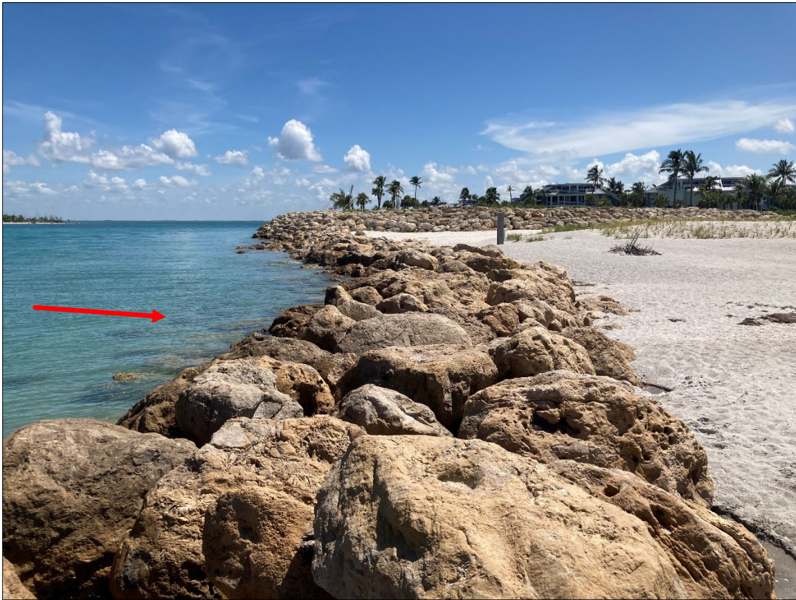
Figure 6. East view of the groin with randomly exposed stones on the northern side of the groin.
